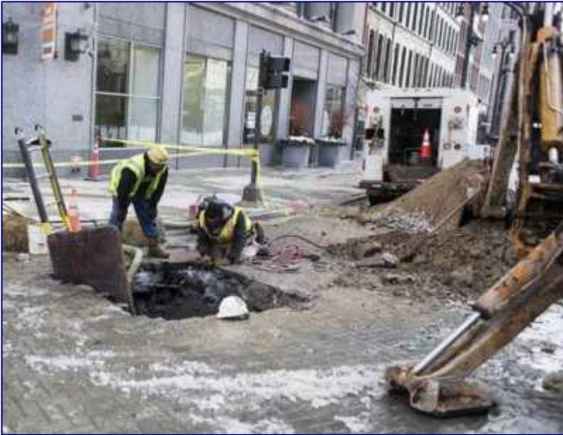
**DWSD workers make repairs using equipment serviced at auto shop, going into manhole.**
